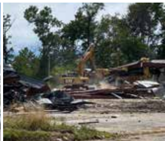
Noble Gas is coming to Orange. Demolition is being completed and construction will start soon.
