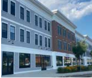
Firelite Commons has been completed and contains 72 housing units plus commercial space.
