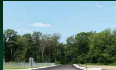
New paving at Fred Wolfe Park.
